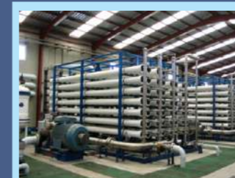
RO/RECYCLING RO PLANTS RECYCLING PRODUCT FLOW 30 M 3 RO PRODUCT FLOW 6 M 3 RO PRODUCT FLOW 12 M 3 RO PRODUCT FLOW 15 M 3
